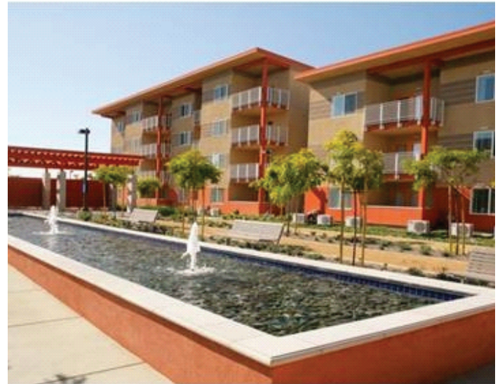
Seasons, LINC Housing: 84 units in Compton, mix of limited-income seniors, seniors with developmental disabilities and formerly homeless seniors
