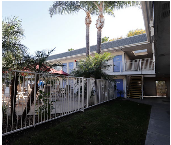
Motel 6 Baldwin Park, converted by the County into housing with 1st Round of Homekey funds
