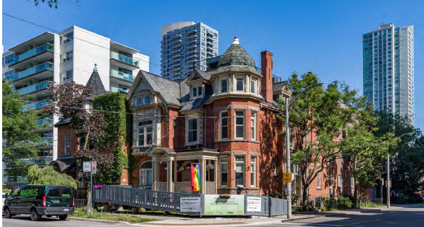
A wheelchair ramp offers accessibility to the Fife House, a historic renovation near downtown Toronto that provides services to people with HIV/AIDS who are also experiencing homelessness.
